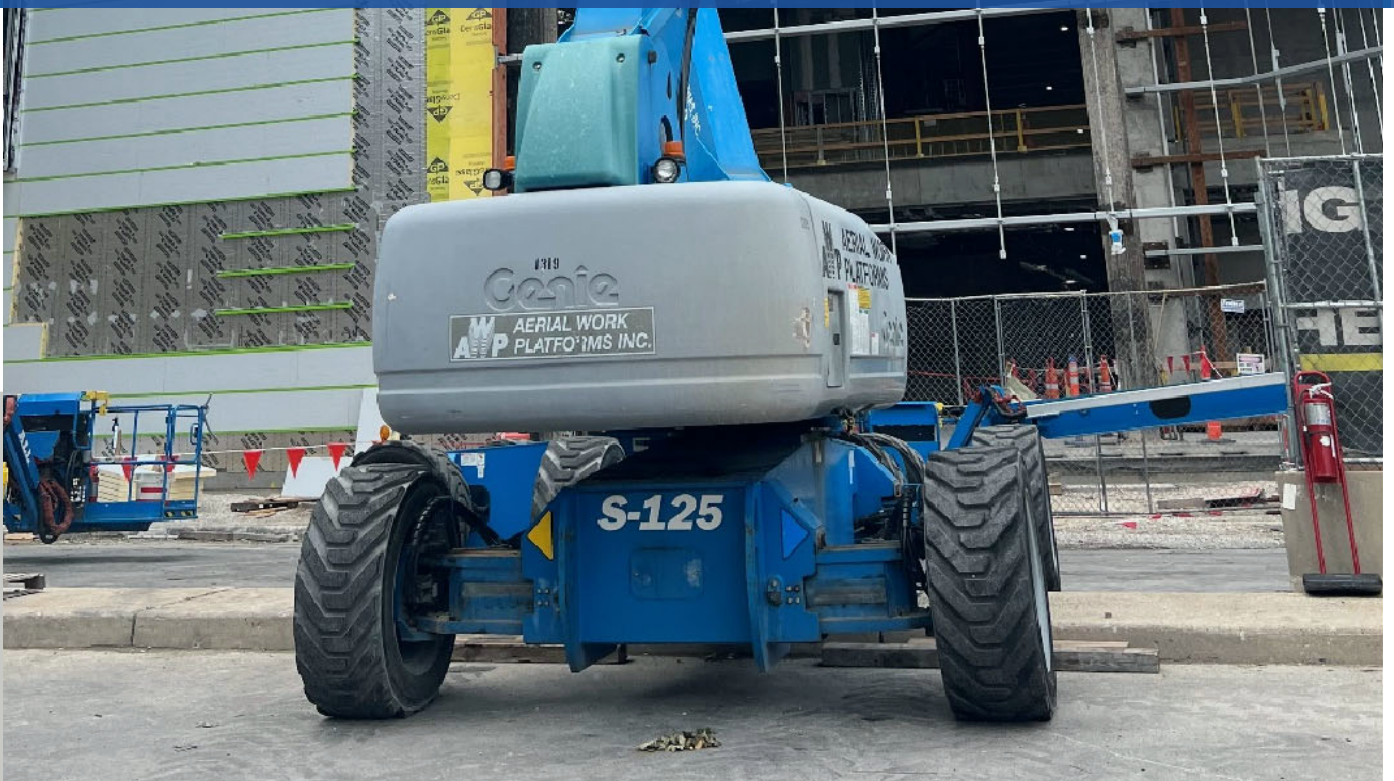
EXTERIOR PANEL PROGRESS – VRP
