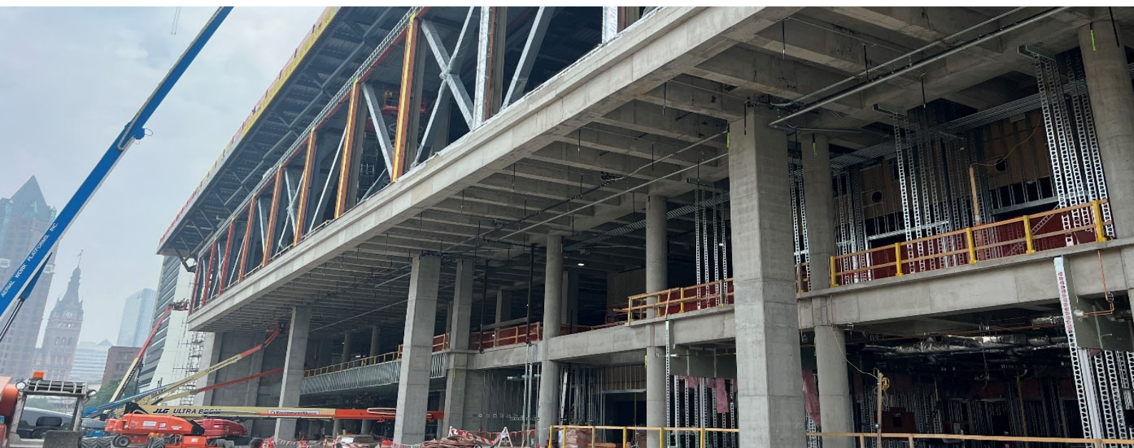
VIEW OF EXTERIOR PROGRESS
