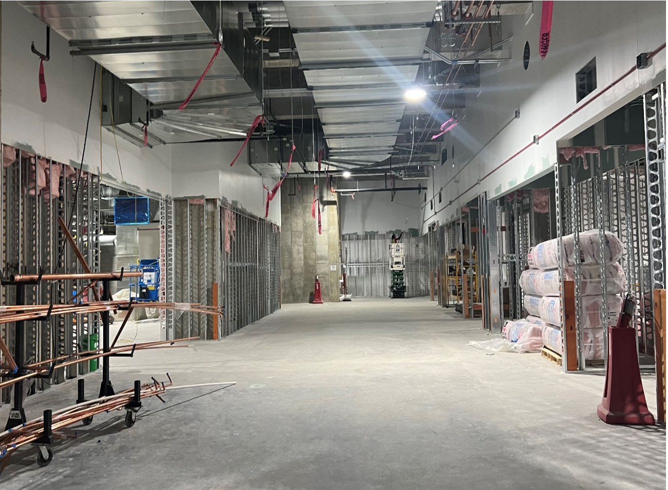
BALLROOM LEVEL – SOUTH WALL FIRE PROOFING AND FRAMING PROGRESS
